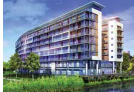
SUTTONS WHARF SOUTH
